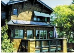
Solar panels are designed as an integral component of the roof to minimize visibility
