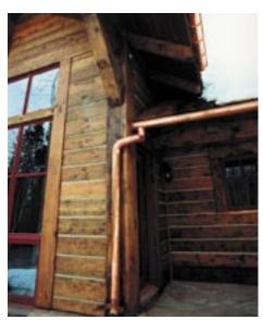
Copper gutter diverts water from overhangs
